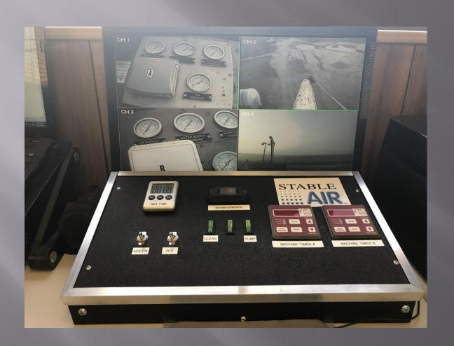
The dispatcher deploys the foam boom and starts the timer which starts the process of foaming the truck. Once the timer shuts off the machine the foam boom is retracted and the driver leaves the area
